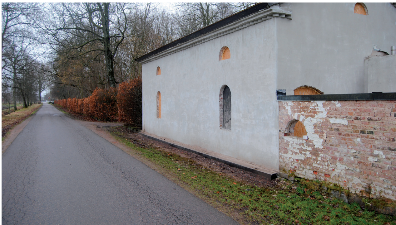
Norra fasaden under renovering.
